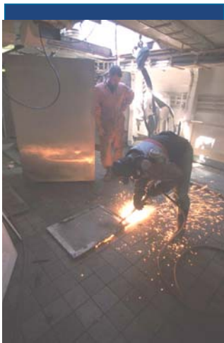
Large holes were cut into her side to allow proper water flow throughout the ship!
